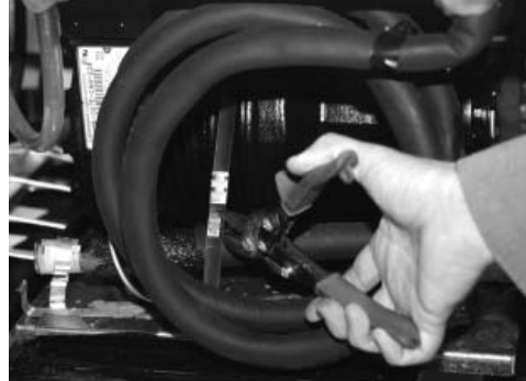
Cutting band that is around compressor
